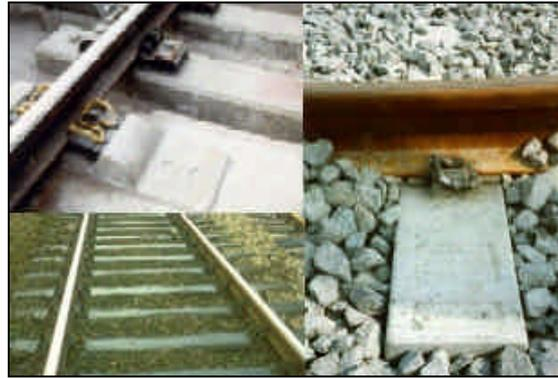
Figure 2 Different types of track support
