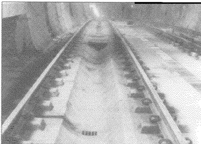
Fig. 6: Edilon Block System with DE fasteners
