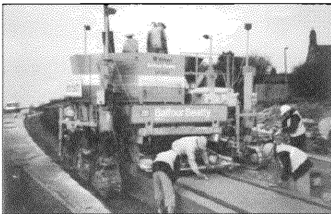
Fig. 11: Slipform paver (Photo: Edilon)
