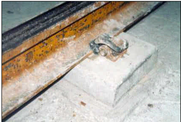
Figure 8 Detail of Edilon Block System with Pandrol fasteners
