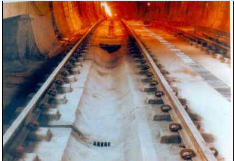
Figure 7 Edilon Block System with DE fasteners
