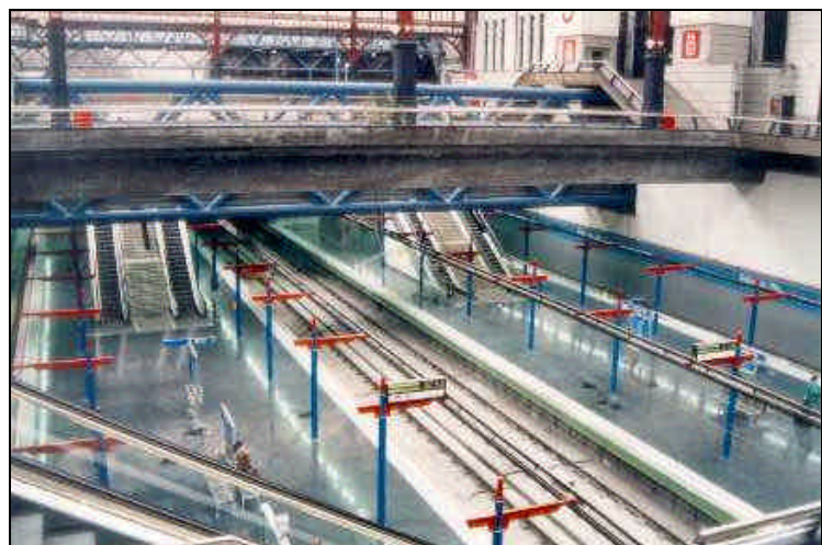
Figure 6 Edilon block track system at Madrid Metro
