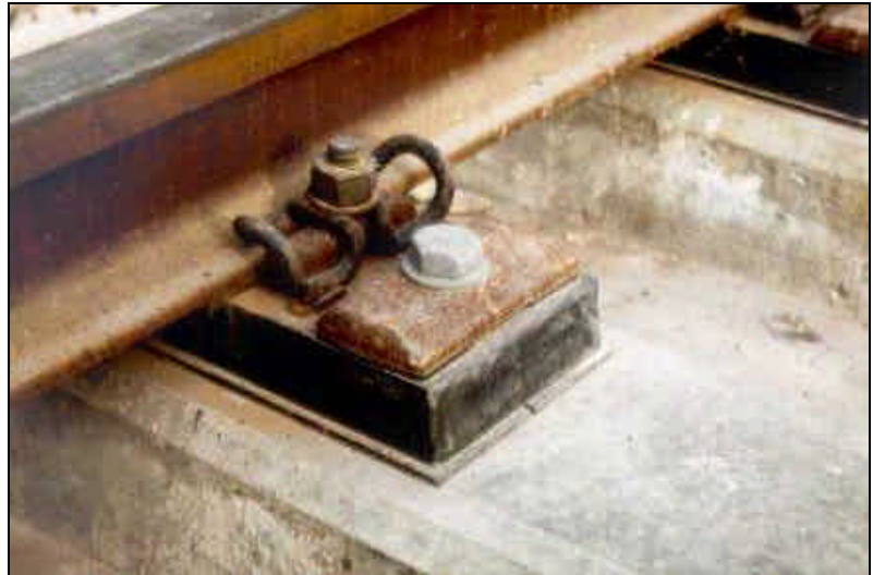
Figure 13 Elastic rail support in track structure, Berlin
