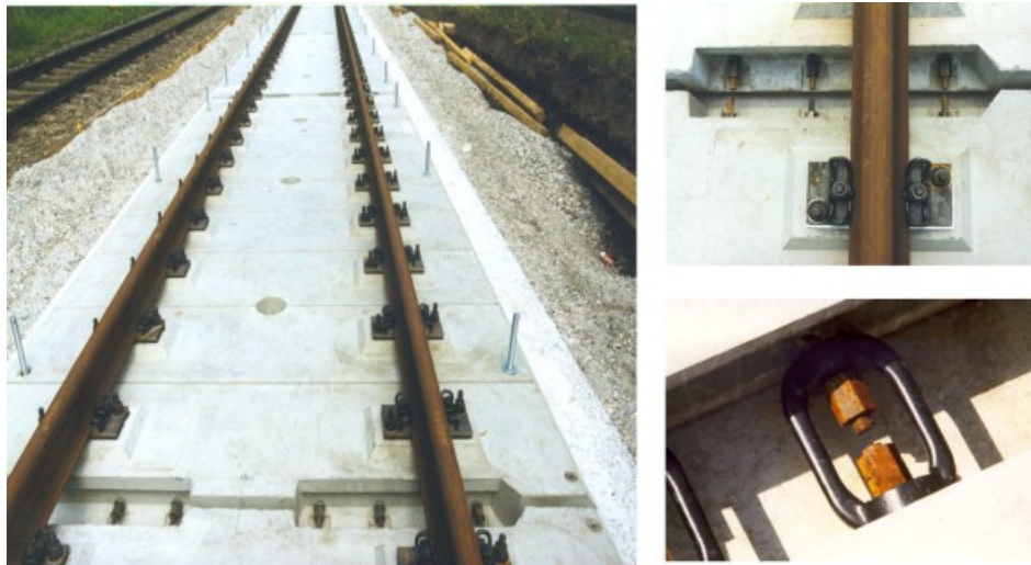
Figure 2.3 Constructional principal of FFB structure
