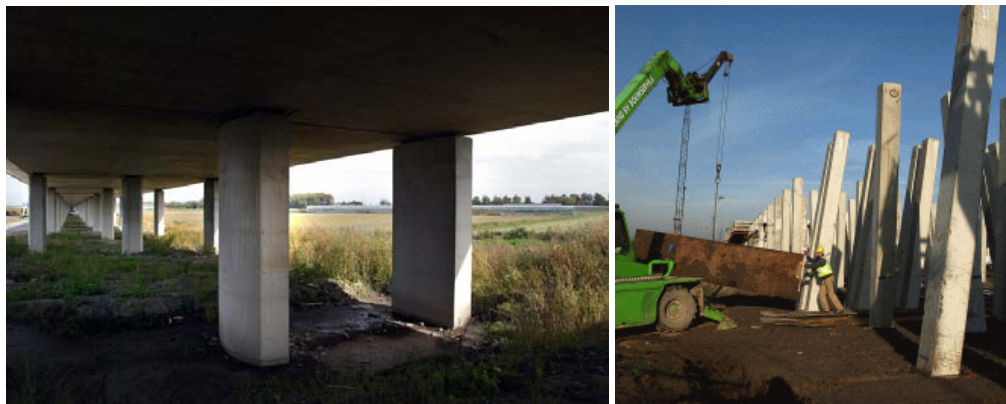
Figure 2.2 Supporting piles of Settlement Free Plates (HSL-Zuid)
