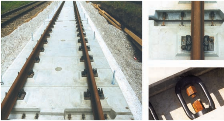
Fig. 3: Bögl slab track system
