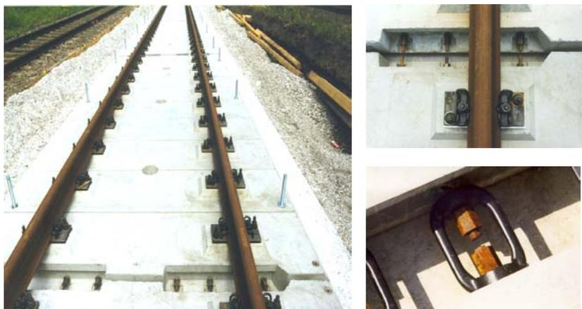
Figure 4 Bögl slab track system
