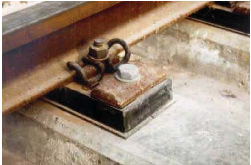
Fig. 9. Elastic rail support in track structure, Berlin
