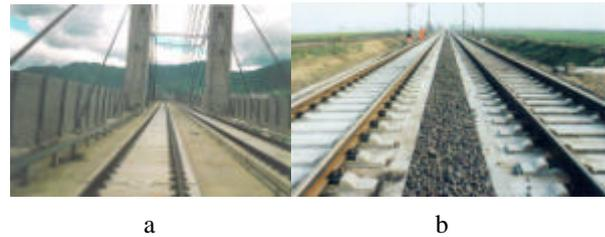
Figure 1 Shinkansen (a) and Rheda (b) slab track structures
