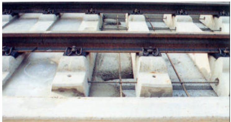
Figure 1 Rheda structure
