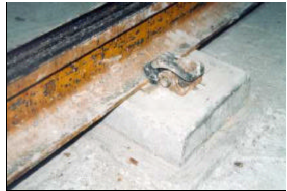
Figure 2 Edilon block track
