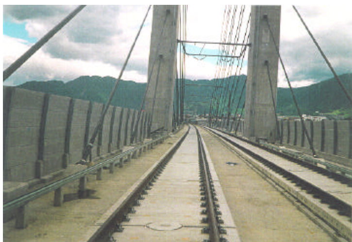
Figure 3 Japanese Shinkansen slab track
