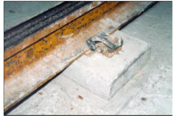
Figure 2 Edilon block track
