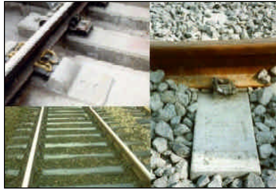
Figure 2 Different types of track support
