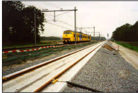
Figure 7 Embedded Rail Structure installation near Best (the Netherlands)
