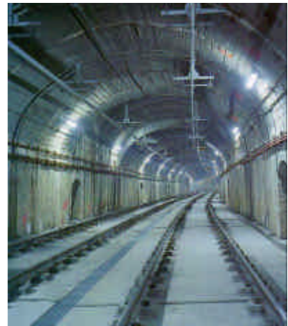
Figure 3. Picture of block track in Madrid Metro (photo AZ)
