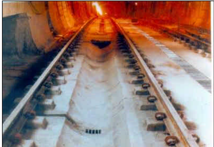
Figure 7 Edilon Block System with DE fasteners
