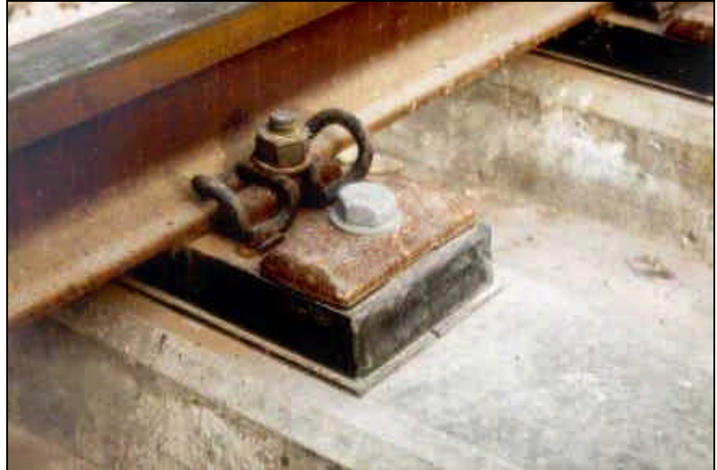
Figure 13 Elastic rail support in track structure, Berlin
