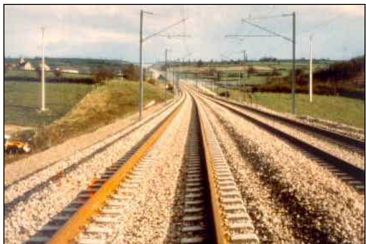
Figure 1 TGV track with twinblock sleepers
