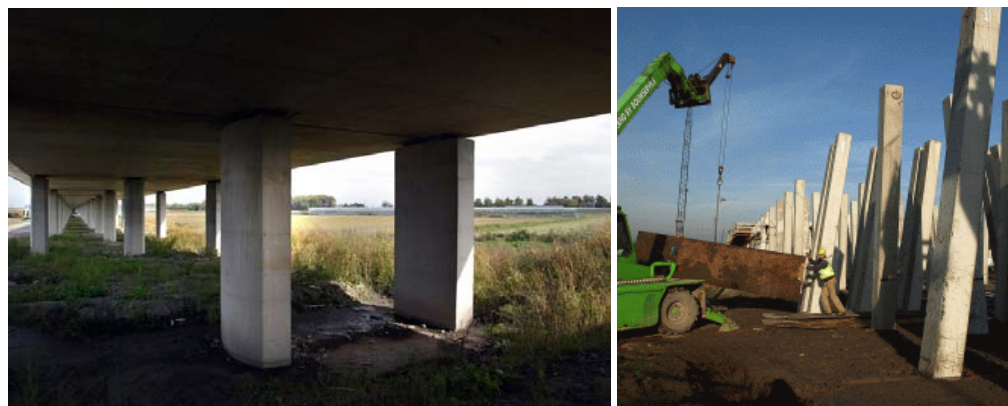
Figure 2.2 Supporting piles of Settlement Free Plates (HSL-Zuid)
