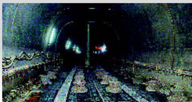
Heitkamp Rail have put their experience of more than 100 years in concrete and railway construction to good use in order to design and to build such mass-spring systems.
