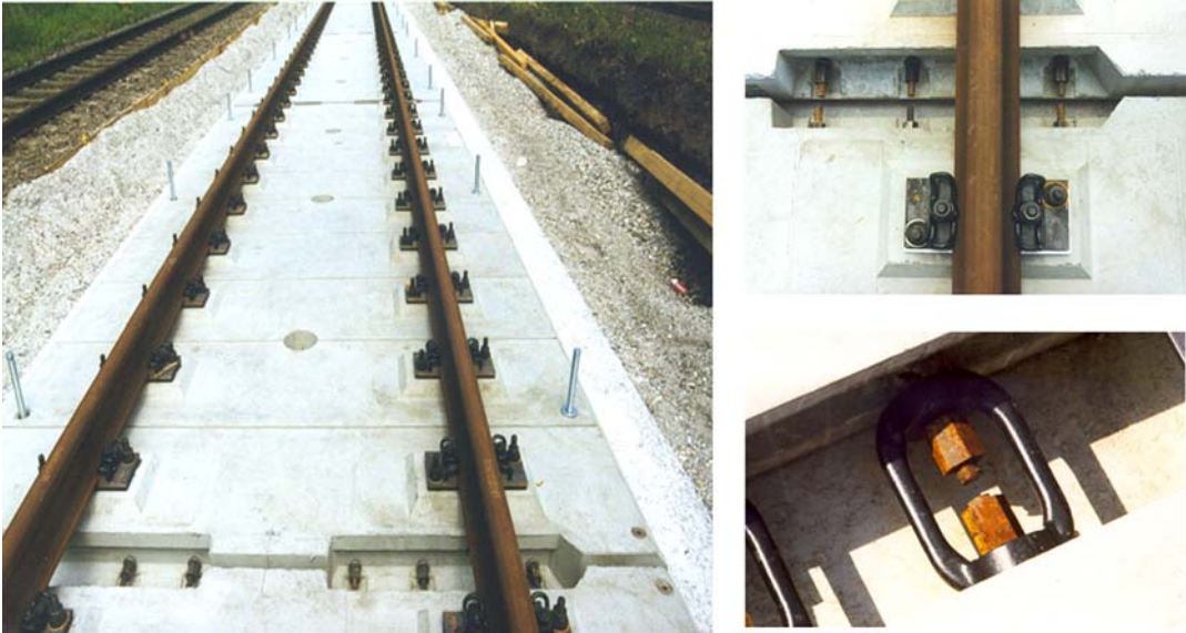
Figure 2.3 Constructional principal of FFB structure
