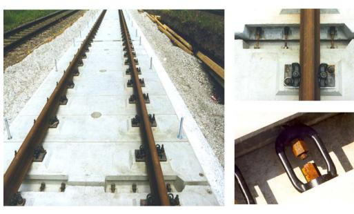
Figure 2.3 Constructional principal of FFB structure
