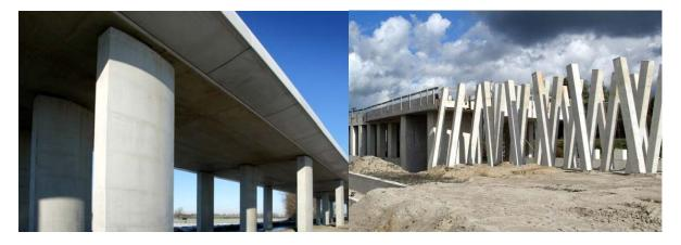
Figure 2.2 Supporting piles of Settlement Free Plates (HSL-Zuid)
