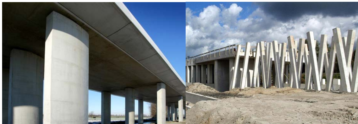
Figure 2.2 Supporting piles of Settlement Free Plates (HSL-Zuid)
