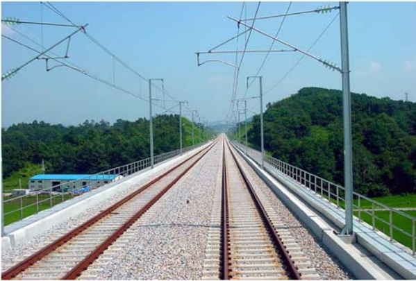
Figure 2 Ballasted HSL track of KORAIL
