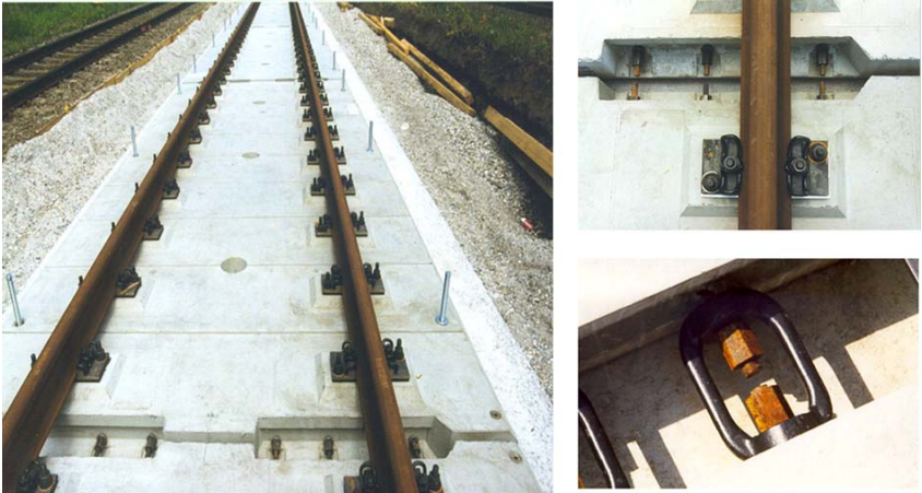
Figure 4 Bögl prefab slab track
