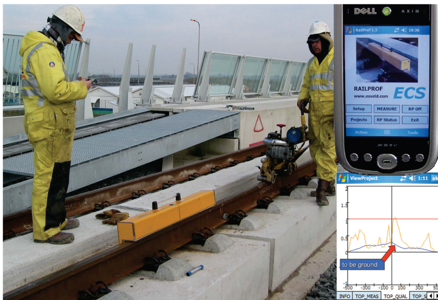
All welds on HSL-Zuid were checked with the RAILPROF
