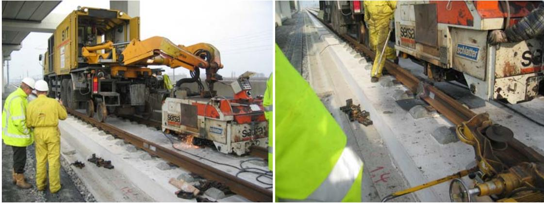
Figure 6 Flash butt rail welding on the HSL-South
