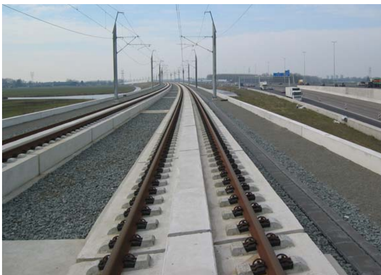
Figure 2 The finished slab track on the Dutch HSL-South
