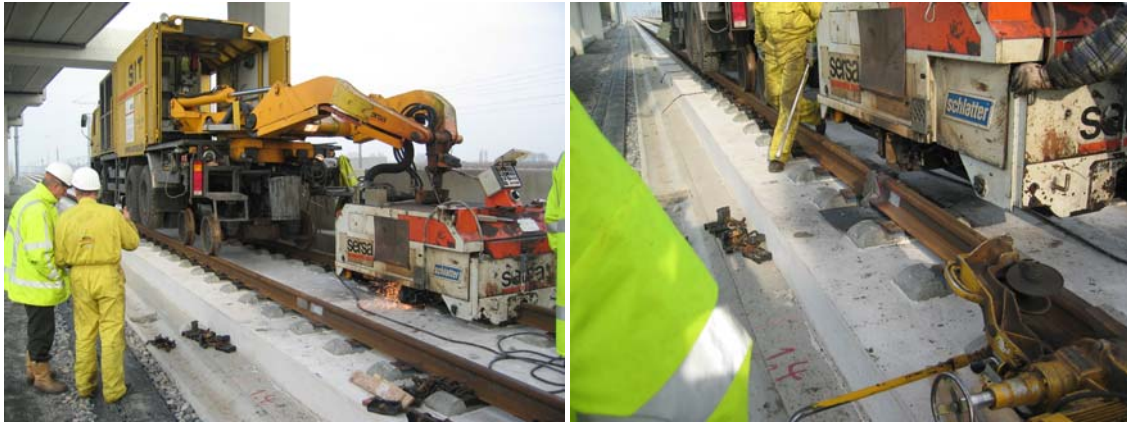
Figure 6 Flash butt rail welding on the HSL-South
