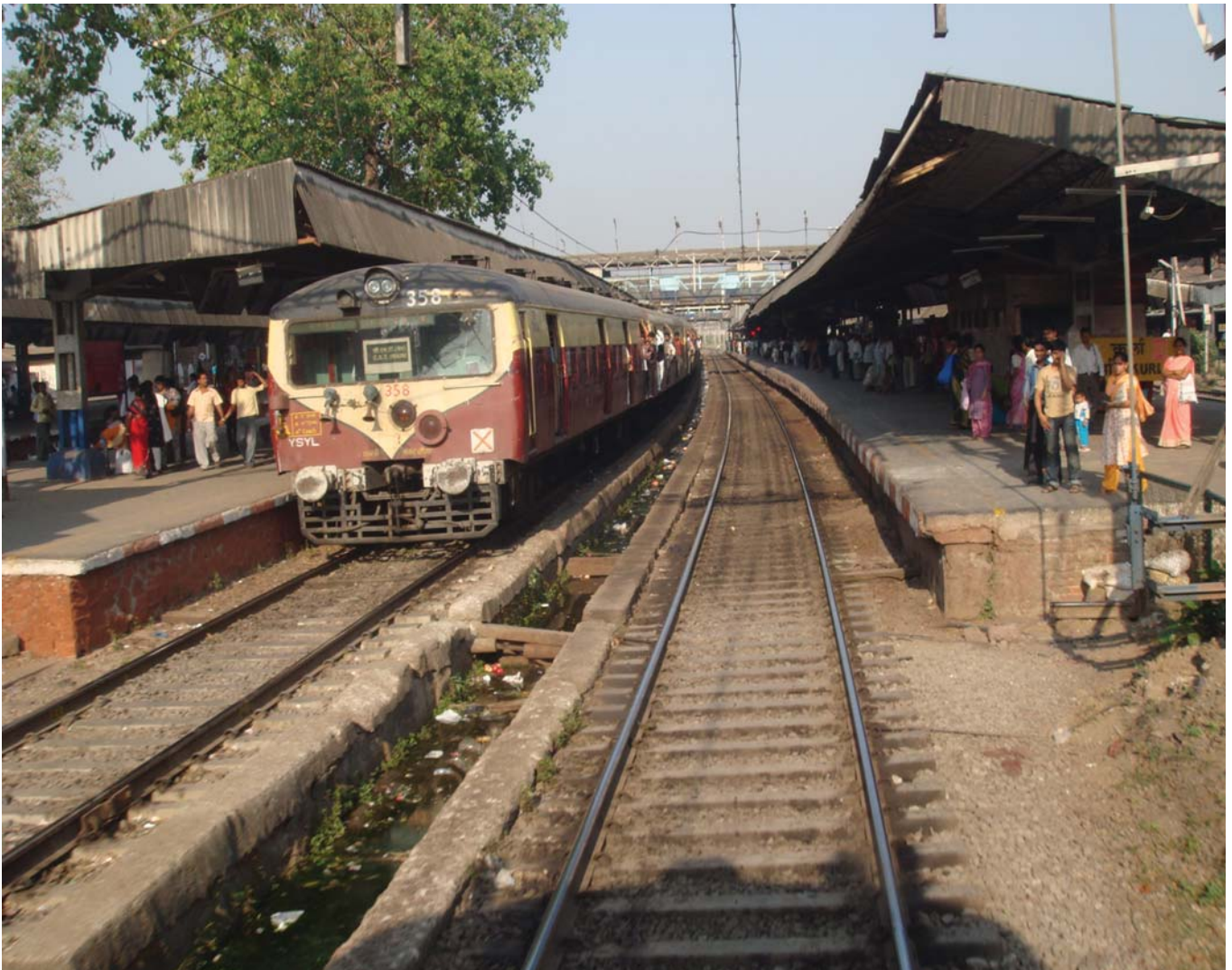
Figure 4: Location on Mumbai Suburban Railways where mechanized - ballast cleaning is impossible
